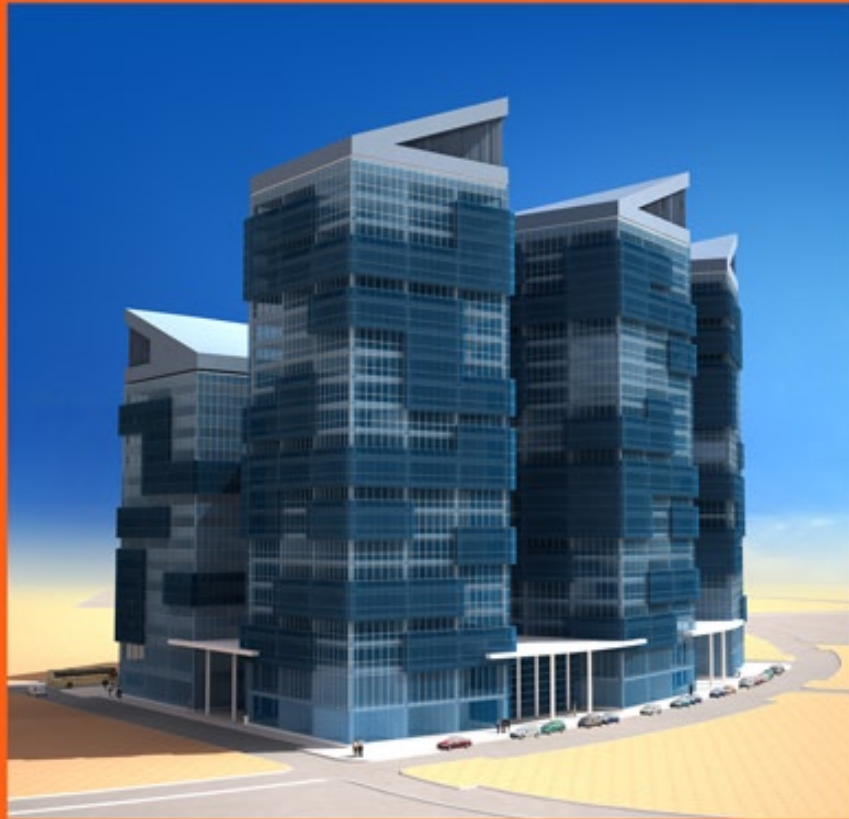
north west corner view
